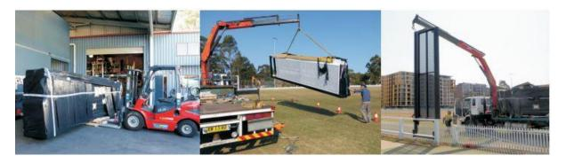
Fig: Eclipse Screen Loading and Offloading.
