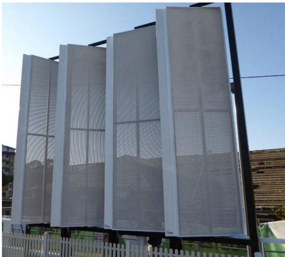
13. When the screen is not in operation, release the latch and rotate the screen 90° and relock the latch.
