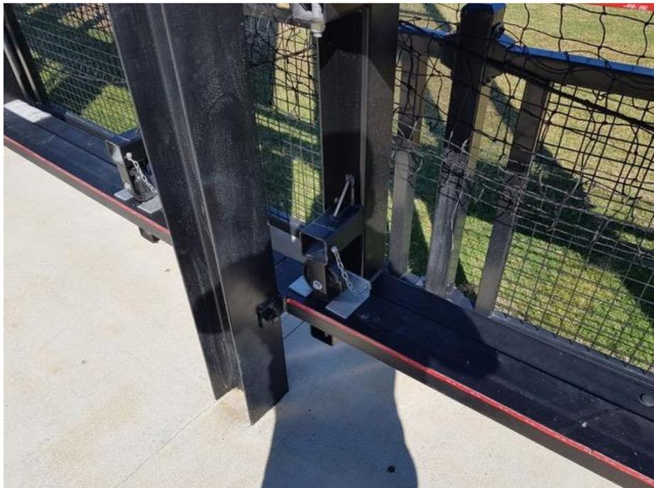
10. Then attach the finger guard to both sides of the upper roller wheel. Use 25MM Hex Metal Screws to screw the finger guard to the side of the upper roller wheel.
