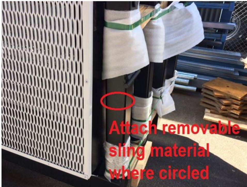
3. Then, slowly lift the sight screen/carriages into place using 2 people to support and guide the carriages onto the track. While lifting, ensure the sling is not slipping to prevent any mishaps or accidents.
