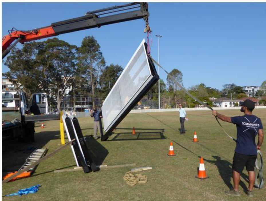
4. Once the sight screen is vertical, slowly position the screen frame with guide rollers into the guide track position. **Caution: Please be careful while placing the wheels onto the track. Do not place the fingers under the channel rail. Serious Injury may occur.**
