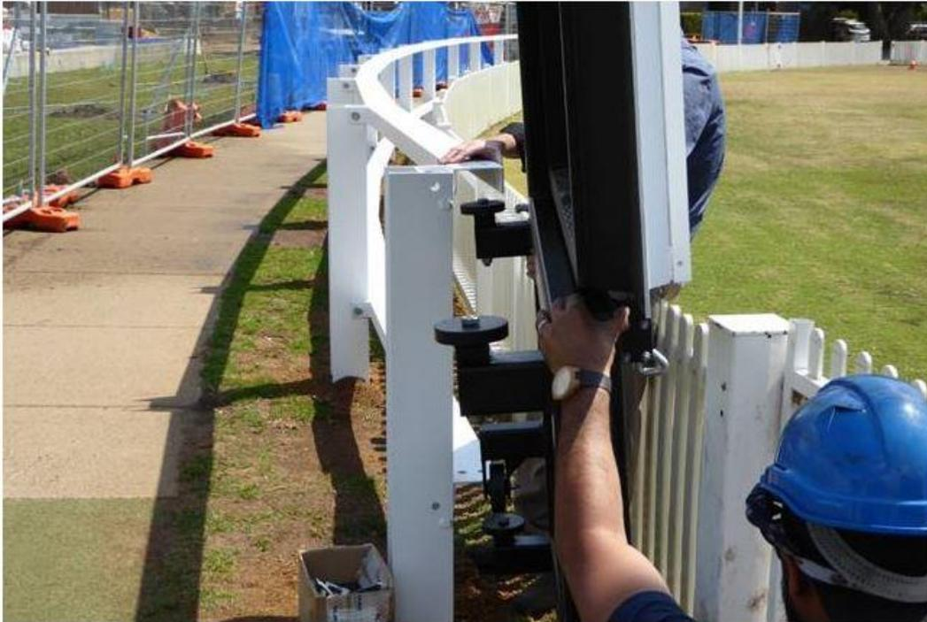
5. Align the guide wheels with the guide track railings and start moving the screen along the track.
